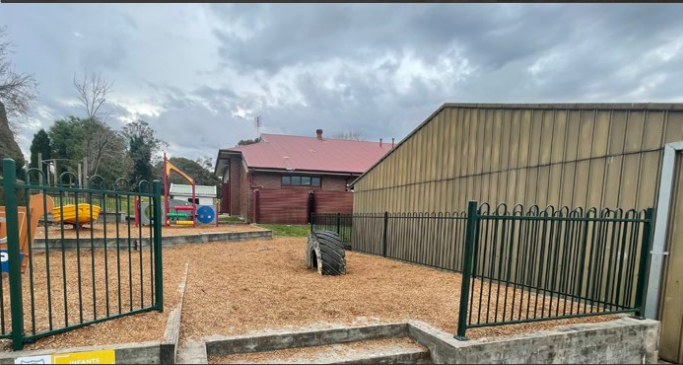
5. EXISTING PLAYGROUND AREA TO BE RETAINED
